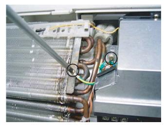
11)Remove a screw fixing the control box cover.
