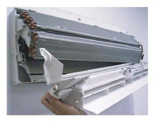
23)Take out the right side of the drain pan,leaving drain hose in cabinet
