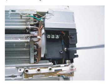
12)Remove the control box cover.
