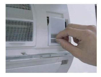
4) Remove the unit-to-unit wiring from the terminal board
