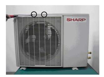
5) Loose 5 screws fixing the front panel.
