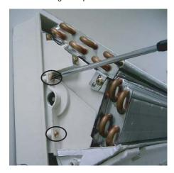
20)Remove drain joint screw.
