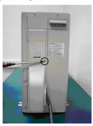
2) Loose 2 screws fixing the terminal cover and 1 screw fixing the cord clamp.
