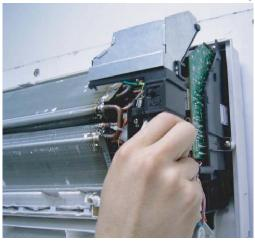
13)Cut the band and take out the sensor from sensor holder.
